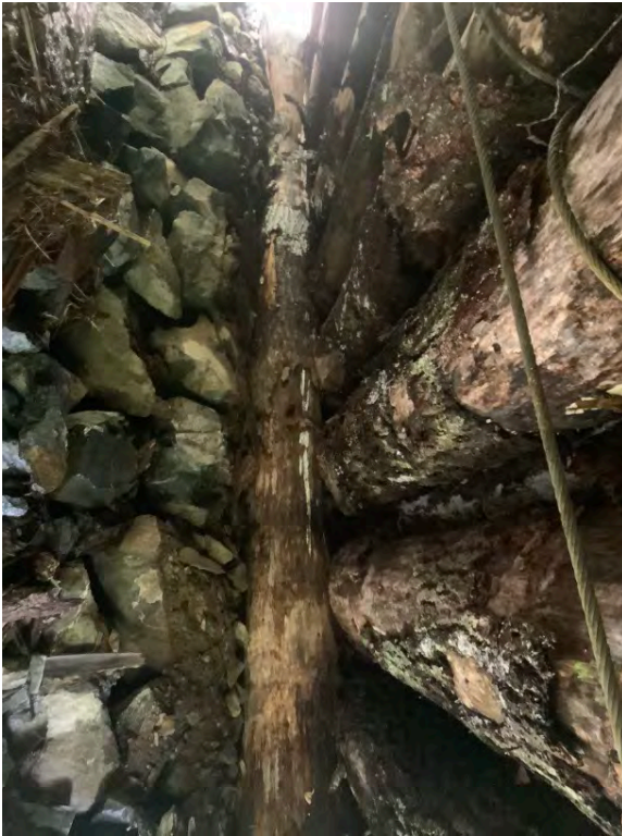
Left Bank Abutment when facing downstream
